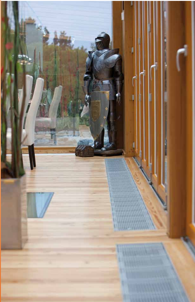
Links: Bodenkanalheizung
